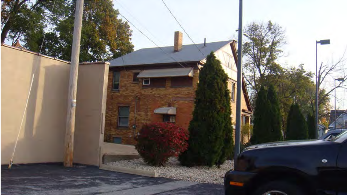
Rear of existing dwelling at 911 Decatur Street
