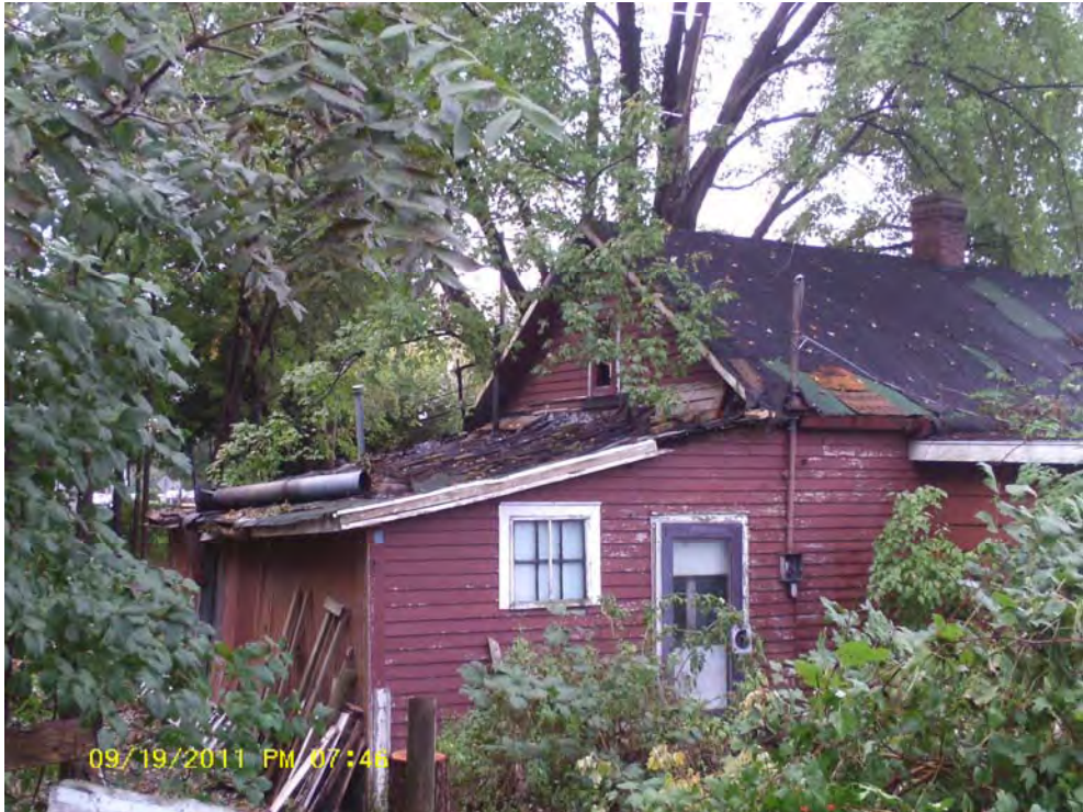
Rear of existing dwelling on 302 Fremont Avenue
