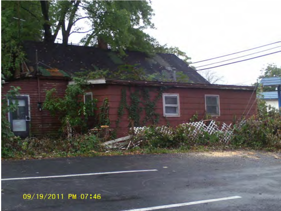
Existing dwelling on 302 Fremont Avenue to be demolished
